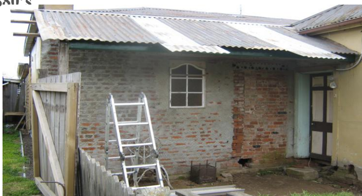
Restoration of verandah is slowly taking shape
